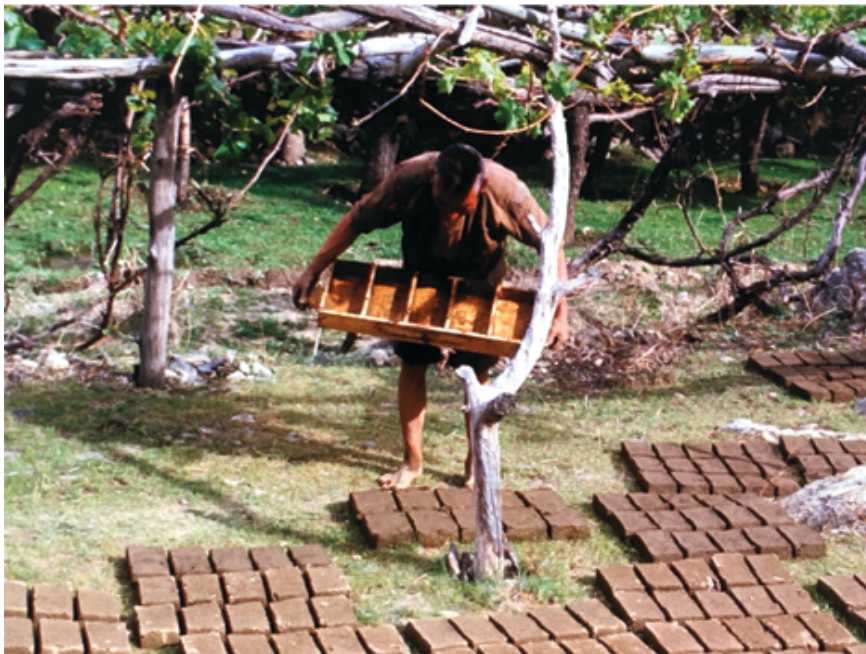
Making the mud bricks for the interior partition walls
